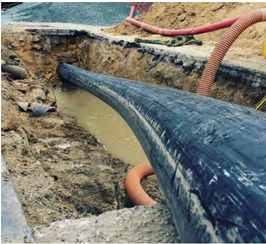
Eight-inch pipe bursting launch pit in Monterey.
