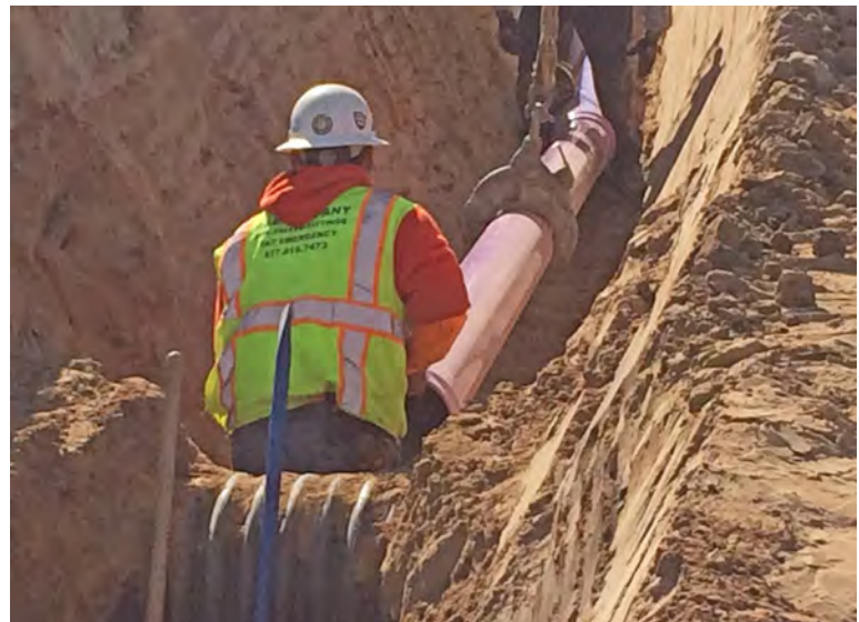
Recycled water main pipeline installation for the East Garrison Development project.
