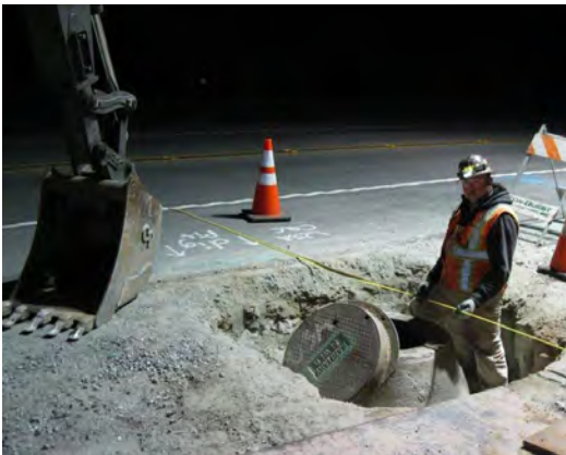
Night work helped minimize impacts to traffic and the local community.
