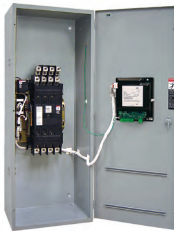
Fig. 4: ASCO Power Transfer Switch rated 600 Amps
