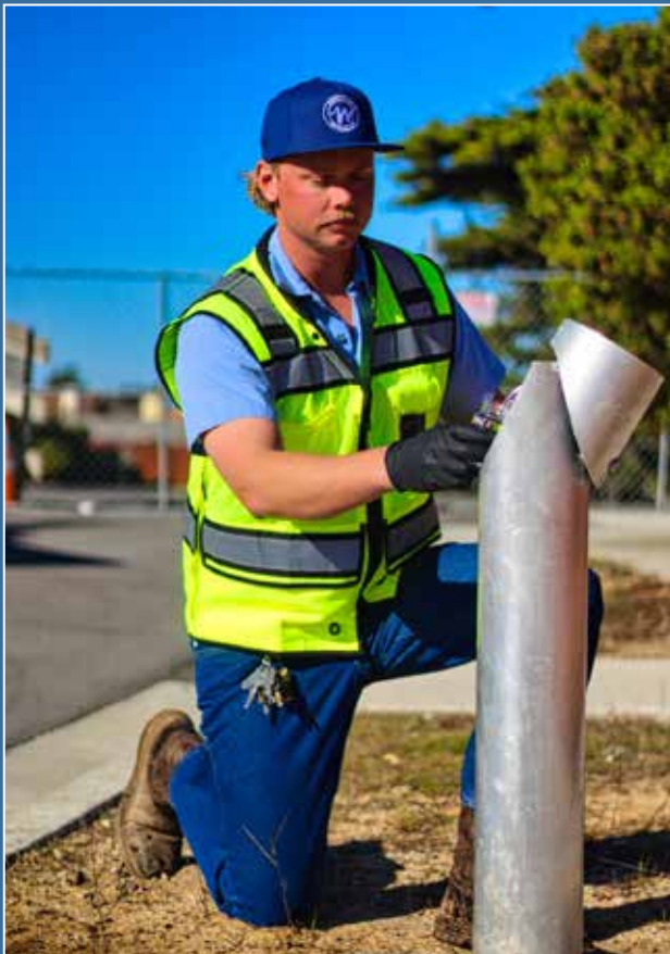
MCWD Operator collecting a routine distribution water sample
