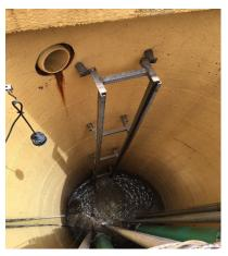
The wet well coating appears to be in good condition, though there is rust bleed below a drain line that is recommended to be recoated. The wet well is 8-ft in diameter and 24-ft deep.
