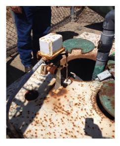
Level control is provided by a float on a vertical rod, which actuates a switch that is mounted above the wet well cover. The level control appears to be in poor condition and in need of replacement.
