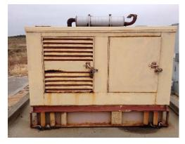
The generator enclosure and exposed exhaust system components are heavily rusted. The subbase fuel tank has minor-to-moderate rust. It is recommended for the generator to be replaced.
