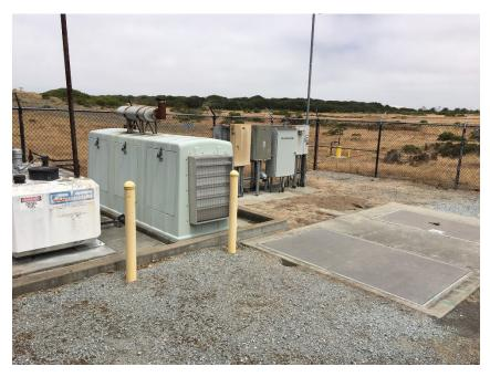
The Reservation Lift Station is a wet well submersible lift station with no building. Valves and pipes on the discharge side are below grade. Electrical cabinets are above grade. The lift station is fenced in.
