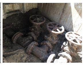
The interior of the valve pit shows signs of cracking and surface damage. The valve pit hatch and the hatch rim are rusty. The bottom of the valve pit is filled with sand. The valve pit should be replaced.
