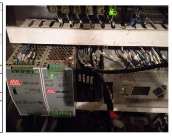
The PLC provides status and alarms to the central SCADA monitoring station via a 2.4GHz radio link, using a Yagi antenna mounted on a rooftop mast. Some components in the SCADA enclosure showed minor signs of rust staining from water, due to rainwater dripping down from the antenna mast. The mast conduit has since been sealed with polyurethane foam, which is also splattered on some of the internal components.
