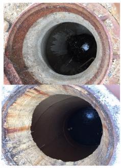
On both sides of the wet well there are manholes. The walls appear to be in good working condition.
