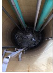
Inside the wet well, the stainless steel pump lifting guide rails appear to be in good condition. The pipes within the wet well also appear to be in good condition and are functioning properly.
