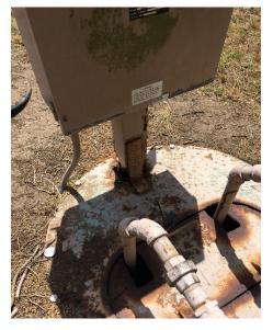
Structural support is inadequate. It is recommended to have a concrete slab for proper pipe support. In addition, the packaged lift station panel appears to be corroded at the base and is in danger of falling over.
