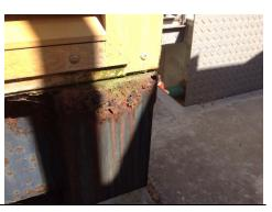
An Olympian model D20P2 diesel engine-generator set, rated at 20 kilowatts/ 25 kilovolt-amps, is located on an adjacent side of the valve pit at the rear of the site. The generator is equipped with a 60-gallon, UL-listed dual-wall subbase tank, and a sound-attenuating enclosure. The generator enclosure and tank have localized areas of moderate-to-heavy rust.
