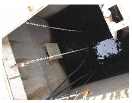
The wet well walls appear to be in good condition. The wet well dimensions are 8-ft long, 8-ft wide, and 11-ft deep.
