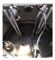
The discharge piping in the wet well shows signs of corrosion.
