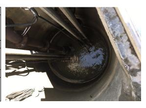
The discharge pipes inside the wet well show signs of corrosion, while the pump lifting guide rails appear to be in good condition.
