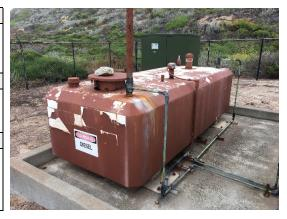
Concrete slabs-on-grade are provided for the generator, fuel storage tank, and outdoor electrical facilities.
