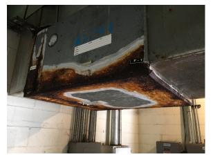
Though the HVAC was reported to be working properly, there appears to be signs of corrosion.
