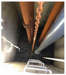
Piping and valves show signs of corrosion both inside the well and on the discharge side (For Photo - See Bypass Pump in Section 4.4.1.) of the pump station.
