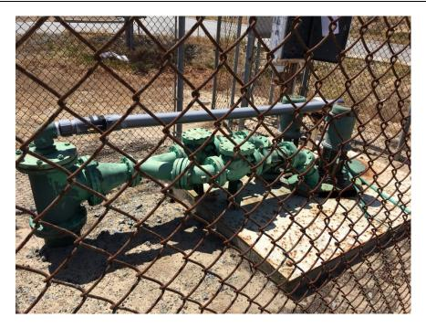
The Neeson Lift Station is a wet well submersible lift station with no building. Valves and pipes are above grade. Electrical cabinets are above grade. The entire lift station is fenced in with limited space.
