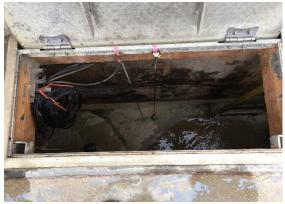
Dimensions of the wet well are 12-ft long, 6-ft wide, and 11-ft deep. The wet well structure appears to be in good condition, but the operator mentioned it is difficult to clean. A larger hatch is recommended.
