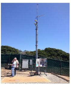
A second antenna, appearing similar to a remote cellular antenna, is mounted at the top of the mast. Cabling from this antenna is routed in underground conduit, and could not be traced. The antenna cable was not observed in any of the equipment enclosures. District personnel also were unsure of its purpose.
