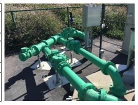
Pipe and equipment support appears to be new and in good working condition.
