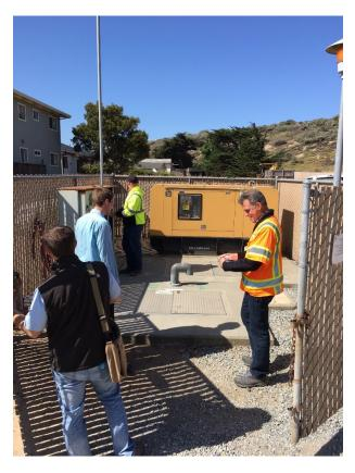
The San Pablo Lift Station is a wet well submersible lift station with no building. Valves and pipes are below grade. Electrical cabinets are above grade. The entire lift station is fenced in.
