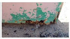
The lower corner of the pump control panel front door is rusted through.
