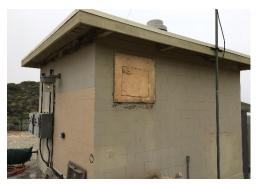
One wall appears to have a boarded up louver or duct penetration with a wood plank and may need to be replaced.
