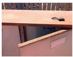
The exterior surface of the NEMA 3R equipment enclosure is weathered and faded with a uniform layer of light rust on the top surface. The edges around the top of the enclosure and around the access doors have moderate rust, but the enclosure is otherwise in serviceable condition.
