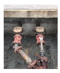
Piping and valves appear to be corroded in the Valve Vault, and are recommended for replacement.
