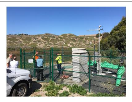
The Dunes Lift Station is a wet well submersible lift station with no building. Valves and pipes are above grade. Electrical cabinets are also above grade. The entire lift station is fenced in.
