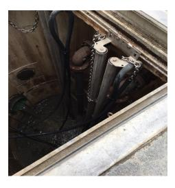
Piping appears to have corrosion issues within the wet well, and it is recommended to be replaced.
