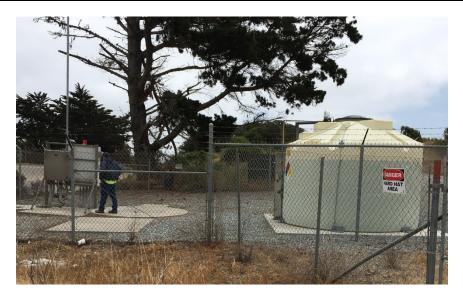
The East Garrison Lift Station is a wet well submersible lift station with no building. Valves and pipes on the discharge side are below grade. Electrical cabinets are above grade. The lift station is fenced in.
