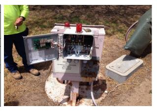
This site is not equipped with the PLC/telemetry package that is present at the other pump stations. The control panel is equipped with two red lights for alarm notification. The presence of an audible device was not noted.
