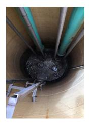
There are two pumps with a maximum capacity of 900 gpm. The wet well water level was lowered for a visual on the pumps. It was confirmed that the pumps were not Flygt models. The operator mentioned that they may have O&M manuals for these pumps. Pumps operate in lead / lag mode.
