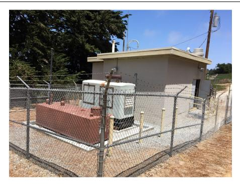
The Gigling Lift Station is a dry pit/wet well lift station with a building. Valves and pipes are in the dry pit below the building. Electrical cabinets are inside the building. The entire lift station is fenced in.
