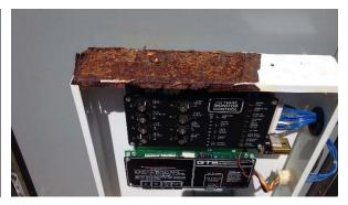
The outer enclosure of the automatic transfer switch is rusted through in two places at the drip edge above the door. Water is dripping inside, causing severe rust to the metal enclosure that protects the ATS control boards. It is a matter of time before the rusted metal no longer protects the control boards from the dripping water.
