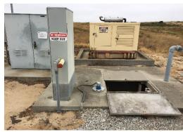
Drawings were not available to show the layout of the site electrical distribution system. Conclusions were drawn from what could be observed above ground. The lift station electrical distribution system is apparently fed from a 12kV distribution system that is owned by the airport, and likely feeds other adjacent equipment installations. The pump station appears to be fed by its own 208Y/120V, 3-phase, four-wire pad-mount transformer.
