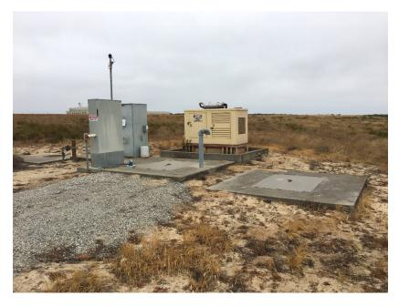
The Fritzche Lift Station is a wet well submersible lift station with no building. Valves and pipes on the discharge side are below grade. Electrical cabinets are mounted at grade. The lift station is not fenced in, though it is inside an airfield, which has perimeter fencing and security.
