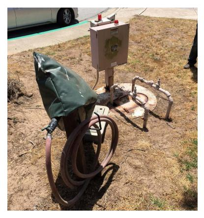
The Hatten Lift Station is a packaged duplex submersible lift station with no building. Valves and pipes are above grade. Electrical cabinets are above grade. The entire lift station has no fence, and is located at the end of the front yard of a residential home. The Hatten Lift Station was construction in 1966, and is controlled by a float system with a capacity of 40 gpm.
