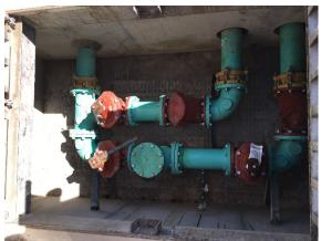
Within the valve pit, a check valve and gate valve are provided on each discharge pipe. The discharge pipes then combine to form a common 6-inch force main leaving the lift station to the west. The valve pit is located behind the wet well at the rear of the site next to the generator, with very little clearance to the side fences.
