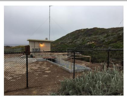
The Ord Village Lift Station is a dry pit/wet well lift station with a building. Valves and pipes on the discharge side are outside the building. Electrical cabinets are both inside and outside of the building. The entire lift station is fenced in.
