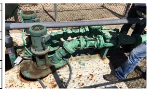
The lift station appears to be in permanent bypass, which is not recommended
