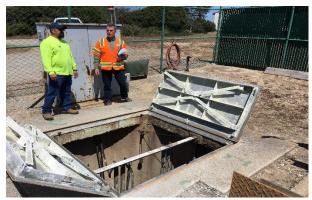
The wet well hatch cover is in fair condition, but fall protection is recommended.
