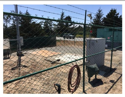
The Imjin Lift Station is a wet well submersible lift station with no building. Valves and pipes are below grade. Electrical cabinets are above grade. The entire lift station is fenced in.
