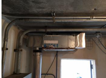
The wet well and dry well vents are connected via a single duct to an exhaust fan that is mounted inside the pump station building. The exhaust fan discharges into the building, not outside. This creates a strong odor problem inside the building, essentially negates the attempt to ventilate the dry well, and potentially creates a hazardous condition inside the pump station building. The ventilation system needs to be redesigned to effectively achieve the pump station's ventilation goals.
