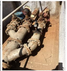
Two new Flygt pumps have a 6-inch diameter ductile iron discharge pipe with a gate valve and a check valve. The discharge pipes combine in a valve pit, and a 10-inch diameter force main conveys flow to the Abrams Trunk Sewer. Only one of the discharge pipes are currently used, thus emergency bypass is not possible. The piping and valves in the valve vault show high amounts of corrosion, and it is recommended to replace all parts within the vault.
