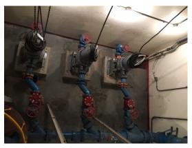
The lift station has three pumps that together run at a maximum capacity of 1.22 MGD (850 gpm), and a TDH of 100 ft. The Flygt submersible pumps were converted to dry pit service. A sump pump in the dry pit has a capacity of 0.07 GPD (50 gpm).
