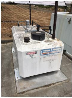
A Convault bulk tank is located next to the generator. Both the generator and tank appear to be in good condition.
