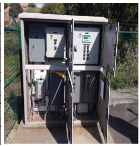
A 100-amp receptacle for connecting a portable generator is mounted to the exterior of this enclosure. Two pump motor starters, a pump control panel, a 480-240/120-volt step-down transformer, and a 240/120-volt lighting panel are located in another fiberglass outer enclosure located on top of the wet well slab. While the
