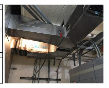
A heating, ventilation, and air conditioning (HVAC) system is also provided to provide ventilation in the below ground areas and to dehumidify the air within the lift station control building (to reduce corrosion and to increase personnel safety). The HVAC system includes a PACE F-1 supply fan, a Baldor 1/3-hp, 530 cfs motor, and a Penn EF-1 exhaust fan with 1/4-hp Marathon motor. Stainless steel ducting draws air from the dry well and
