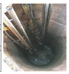
Inside the wet well, the stainless steel pump lifting guide rails appear to be in good condition.
