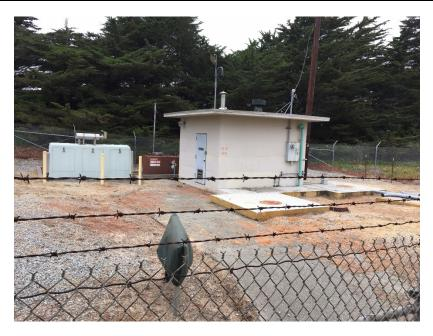
The Booker Lift Station is a dry pit/wet well lift station with a building. Valves and pipes on the discharge side are below the building. Electrical cabinets are both inside the building. The entire lift station is fenced in.
