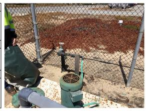
The domestic water hose bibb within the fence did not have a backflow prevention device accepted by the California Code; this was corrected as of the 2005 Wastewater Collection System Master Plan.
