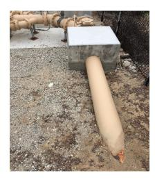
In general, piping and valves appear to be adequate. There does, however, appear to be corrosion at the end of the discharge line, and it is recommended to recoat or replace this section. The extent of exterior corrosion on the pipe is unknown beyond the limits shown in the photo above.
