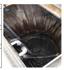
The wet well appears to have a liner rather than coating. No issues observed. Wet well dimensions are 8-ft in diameter and 18-ft deep.
