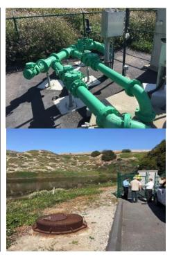
Piping was replaced from the flange out of the wet well up to the ductile iron force main discharge at the intersection nearby. The original pipe routing went up to the old treatment plant, and came back down the hill to a gravity feed. When two pumps were on and stayed on too long it would end up flooding a cleanout near a residence, through the lateral. The piping was rerouted through check valves to a manhole approximately 40 feet near the wet well, which adds capacity.
