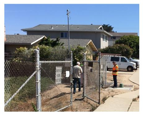
The Crescent Lift Station is a wet well submersible lift station with no building. Valves and pipes are below grade. Electrical cabinets are above grade. While the electrical cabinets are fenced off, the wet well and valve pit are located outside the fence near a residential sidewalk.
