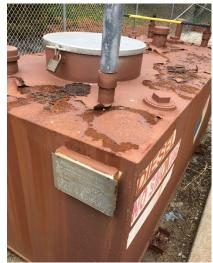
The generator is reported to have engine valve problems and to not be in operating condition. The 250-gallon bulk diesel fuel tank site is heavily rusted. These elements should be replaced.
