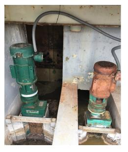
Prior to being converted to a lift station, the Ord Village facility was a wastewater treatment plant. Two open influent channels enter the lift station wet well. Each influent channel is fitted with a Muffin Monster comminutor. The comminutors have 3-hp electric motors with 18-inch helical stack cutters to grind solids into smaller portions for easy passage through the pumps. One of these is highly corroded and is recommended to be replaced (see photo above).
