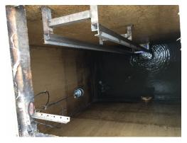
The coatings on the wall appear to be in good condition. Wet well dimensions are 13-ft long, 6-ft wide, and 20-ft deep.
